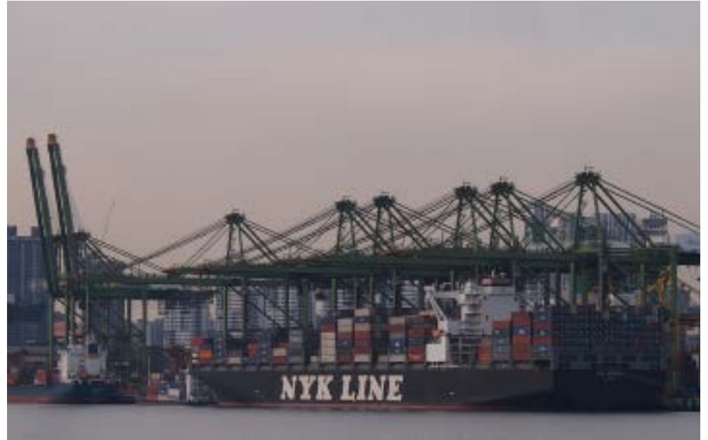
Shore support infrastructure
